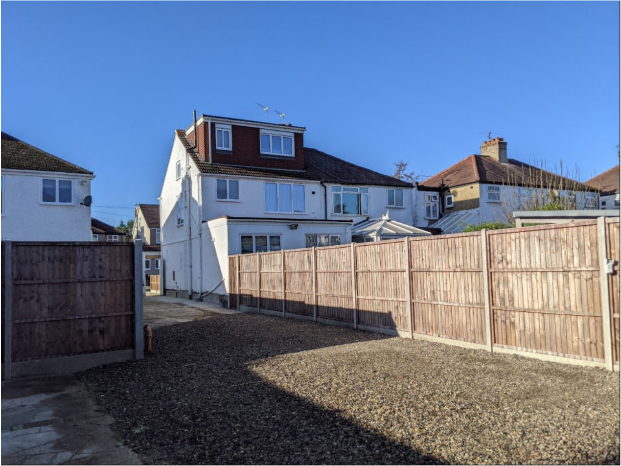
Site Boundaries and Existing Storage Unit on Site boundary and garage.
